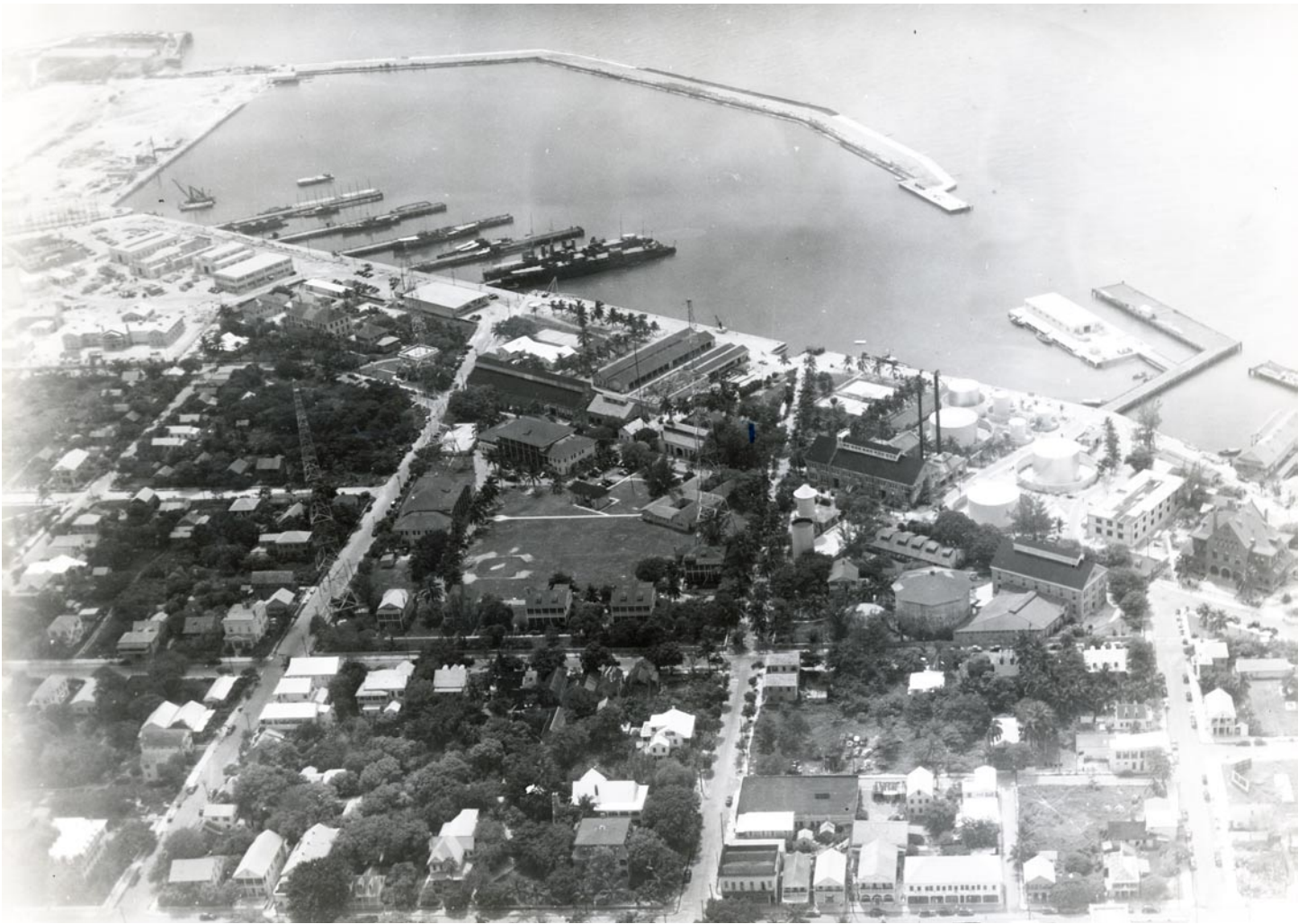
The Key West Naval Station in the late summer 1941. The steel framework of the cradle of the large marine railway that was nearing completion can be seen at the southeast corner of the sub basin (extreme left). To the right of the cradle, a crane on a barge floats over the submerged portion of the rails. This is one of the sites where Henderson Renfroe is believed to have worked as a diver doing underwater welding. Photo credit: Monroe County Library.
