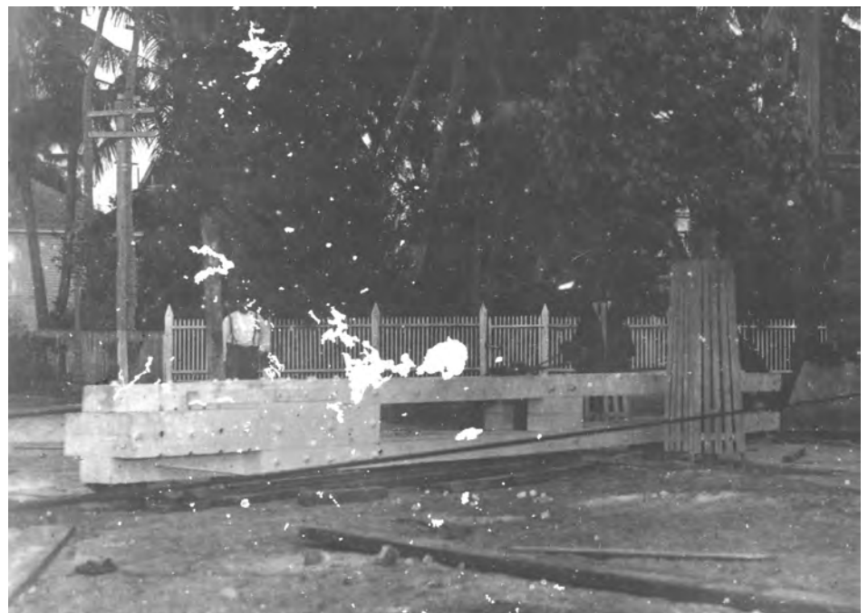
Each segment of the wooden towers was massive and extremely heavy. This close-up shows the large timbers used and how they were bolted together. Note the size of the man relative to the timbers comprising the segment. Photo credit: Wright Langley Archives.
