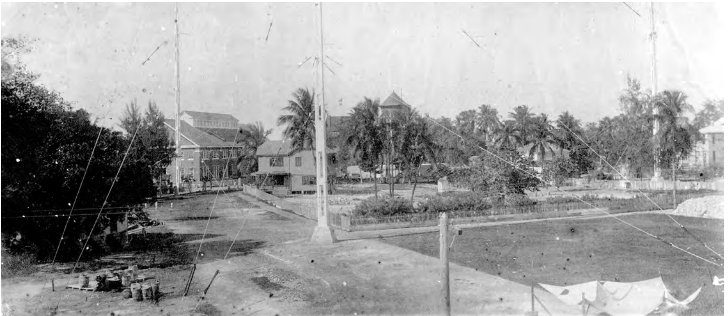
This view (arrow 6 on page 4) was taken from the second floor porch of the two-story house at the corner of Eaton and Thomas Streets. The towers were about three feet square at the base and tapered to one foot square at the top. Photo credit: Wright Langley Archives.
