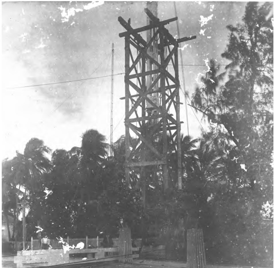
The American De Forest Company used this hoisting rig in 1914 to assemble pre-fabricated segments together to form a tower. In the view above, the hoisting rig supports the segments already joined together while another segment lies on the ground ready to be loaded into the rig. A completed tower can be seen in the background. Photo credit: Wright Langley Archives.
